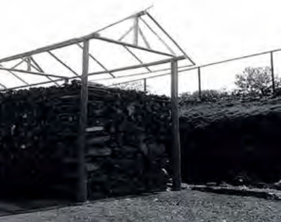
The shed built which has a high and steeply angled roof of transparent polythene and a vacant space between the stacks of firewood and the roof was constructed during the year using local skills and has enabled WATA to achieve the desired outcome.
